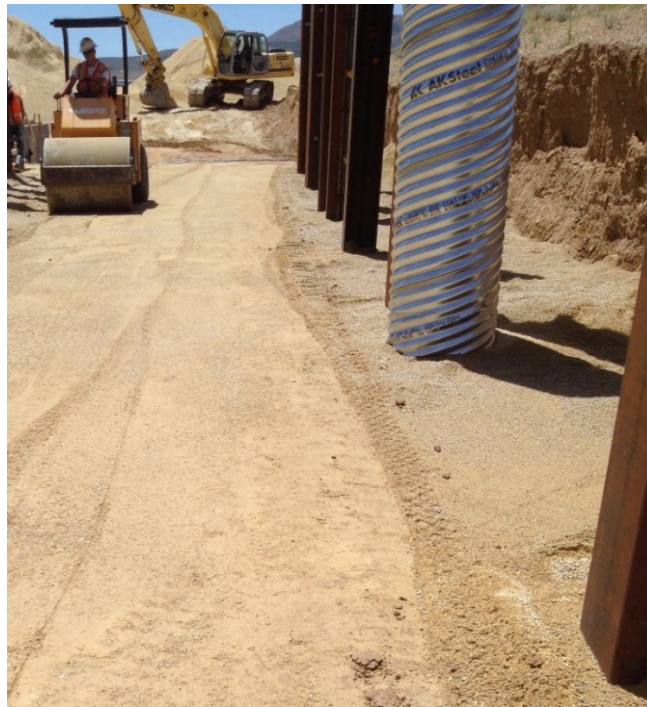
Figure 3-6: Phase 1 compaction
